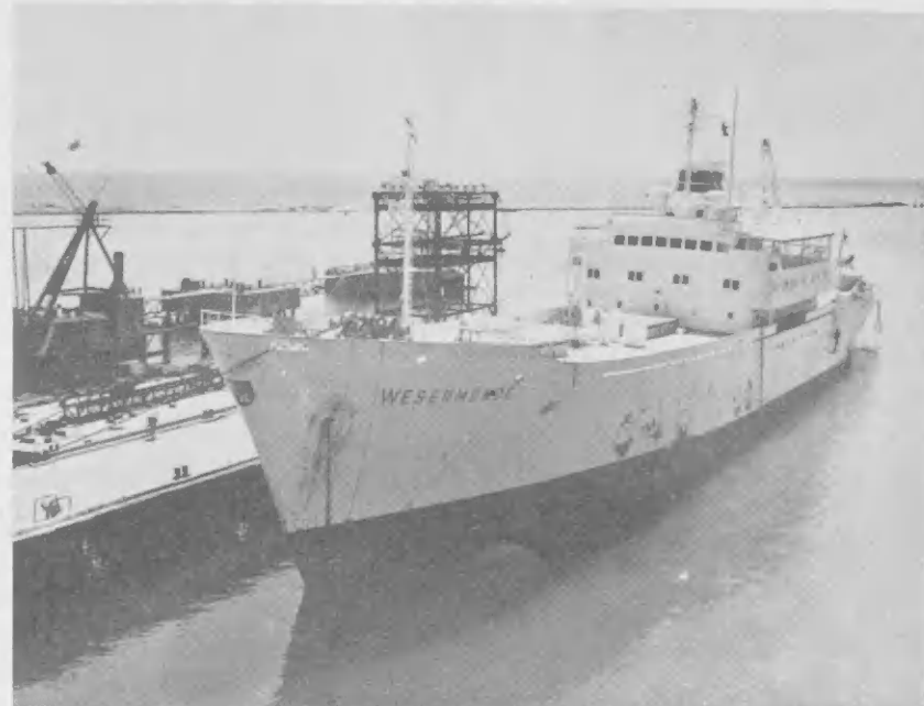
LAST SHIP to call at No. 4 Finger Pier was the Wesermunde, German flag ship. She sailed at 0600 Sept. 15 after which the pier was taken out of service for dismantling.
